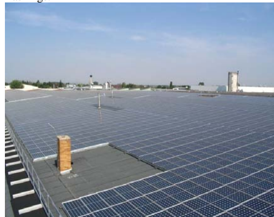
Figure 12: SOLRIF roof to protect a tar-bitumen roof sheet. With a tight lower roof slope angles of 10° are possible.
