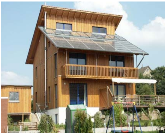
Figure 11: Combination of SOLRIF with thermal solar collectors.
