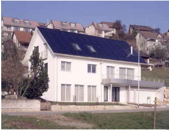
Figure 9: Single family house completely covered with SOLRIF.
