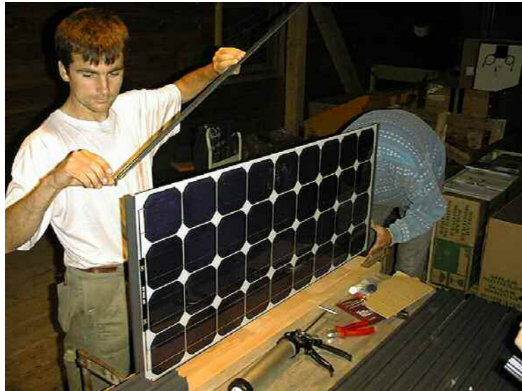
The picture shows a team framing PV laminates.
