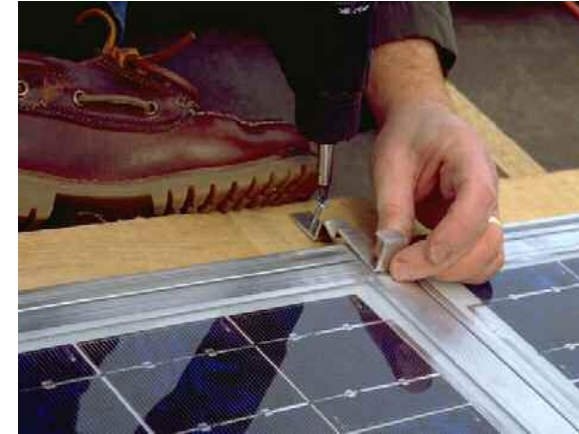
Step 7: Mount the next row of clamps above the installed modules. Use a simple form (piece of wood or similar) to find the correct vertical position for the stirrup. (This is necessary for later single module removal.)
