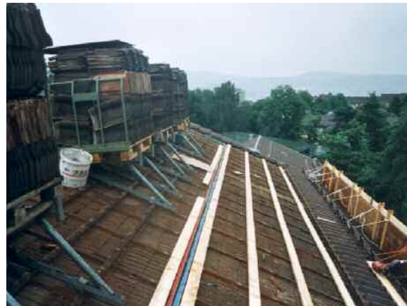
Step 3: Install the new battens according to the layout for the PV modules, install the cabling channels and lay down the string cables.
