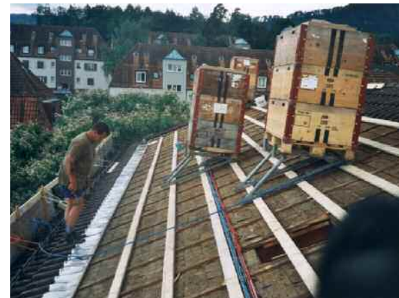
Step 4: Mount the bottom lead or zinc sheets or any other bottom flashing.
