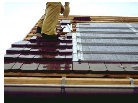
Step 11: Install and fix the vertical flashing.
