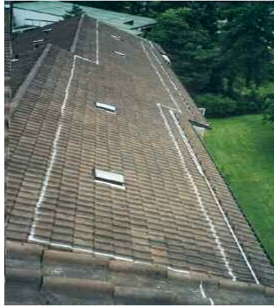
Step 1 (renovation): Mark the shape of the new PV field on the roof.
