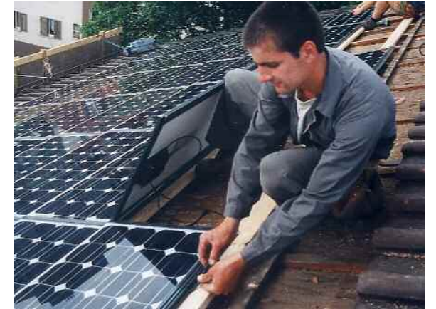
Step 8: Connect the modules according to your cabling plan.
