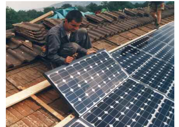
Step 10: Lay down the module. Repeat step 7 to step 10 until all modules are installed.
