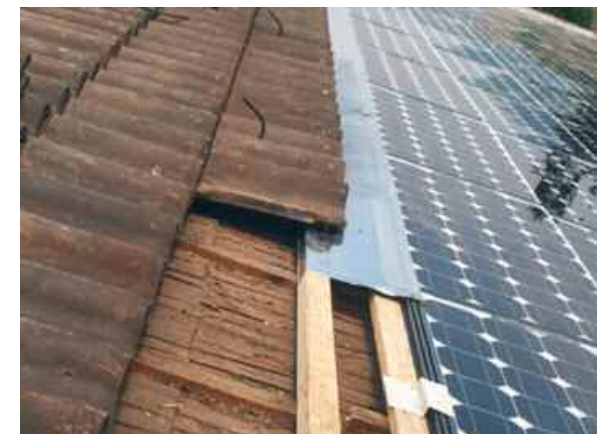
Step 12: Install and fix the flashing at the top and insert the overlapping tiles.
