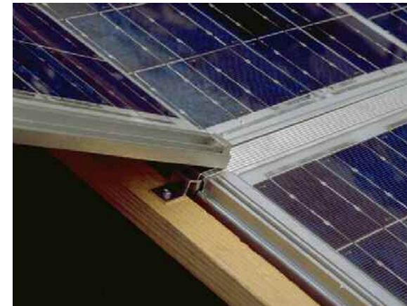
Step 9: Insert the lower module edge into the clamp.
